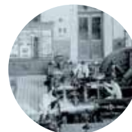
Steam & Gas Turbine Aurel Stodola
